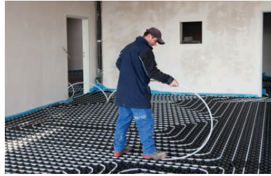
In radiant heating, the boiler circulates heated water through flexible tubing, which can be installed under floors and behind walls. It can even be installed outside — under walkways, patios and driveways to melt snow and ice.
